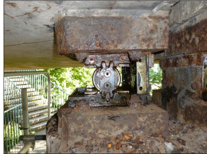
Bearing A1 – South Elevation
