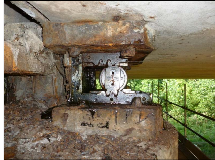
Bearing B1 – North Elevation
