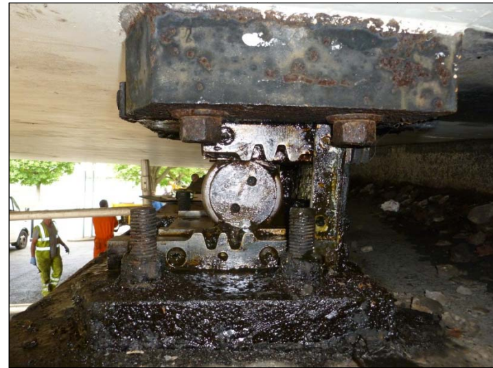
Bearing C – Roller Guide Removed For Ultrasonic Testing
