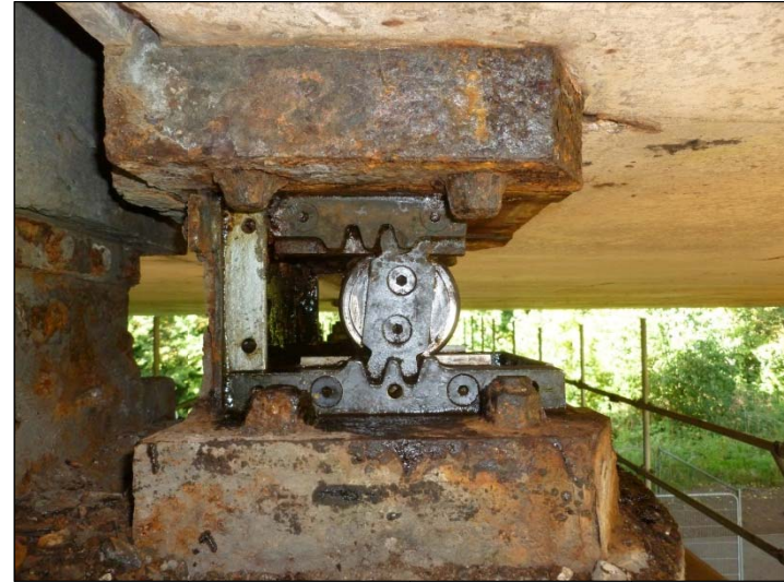
Bearing A1 - North Elevation
