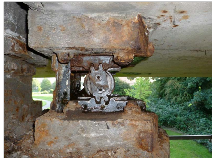
Bearing A2 - South Elevation
