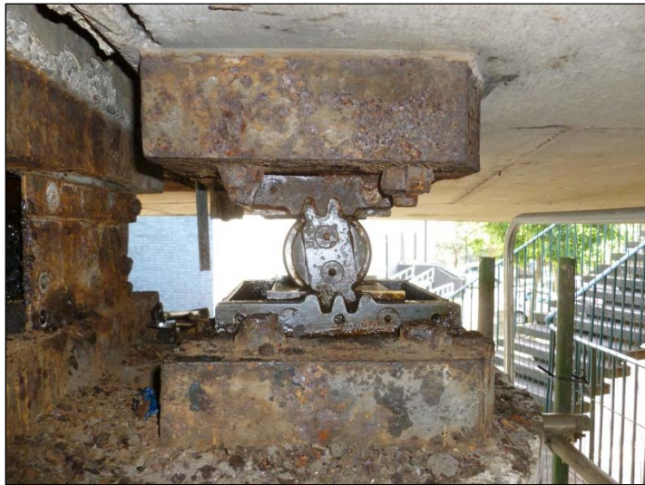
Bearing C1 – North Elevation
