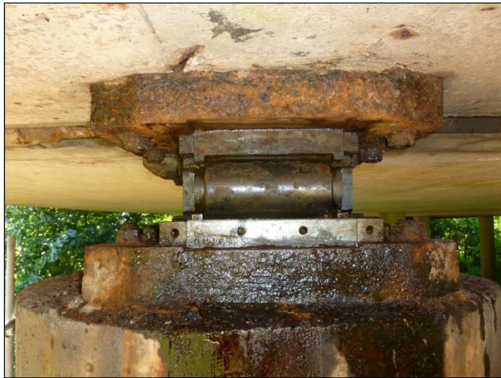
Bearing A1 with Grease Box Removed
