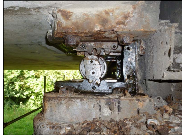
Bearing C2 – North Elevation
