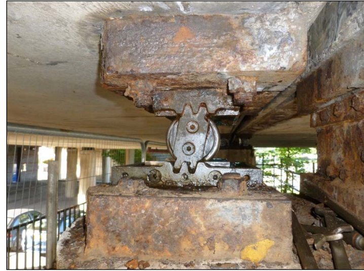
Bearing C1 – South Elevation
