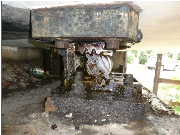
Bearing C – North Elevation
