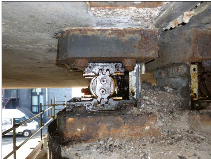
Bearing B2 – North Elevation
