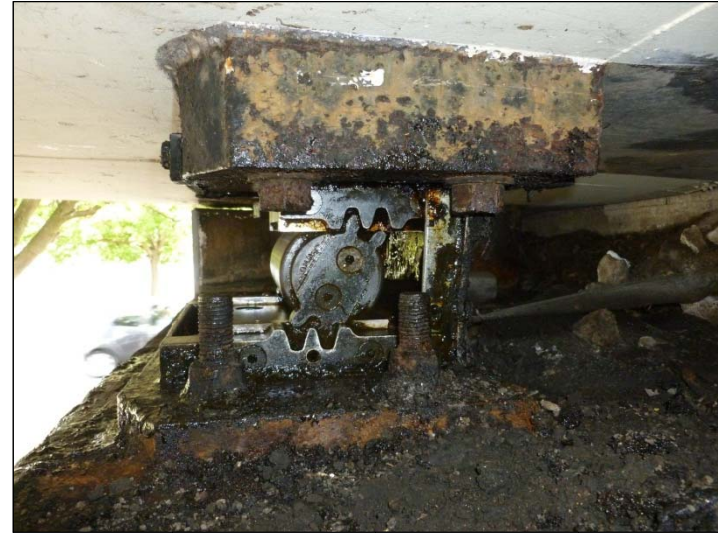
Bearing A – South Elevation
