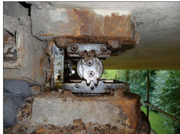
Bearing B2 – South Elevation
