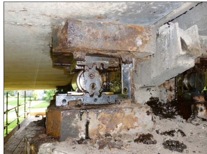
Bearing C1 – South Elevation
