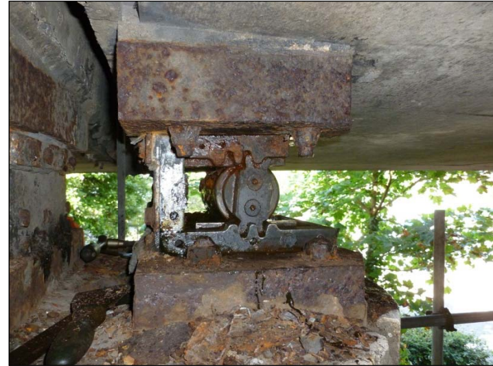
Bearing A2 – South Elevation
