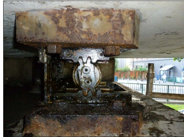
Bearing B – North Elevation
