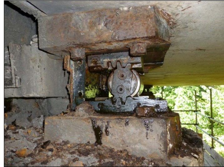
Bearing C1 – North Elevation
