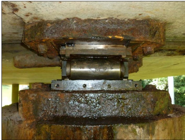
Bearing D1 with Grease Box Removed
