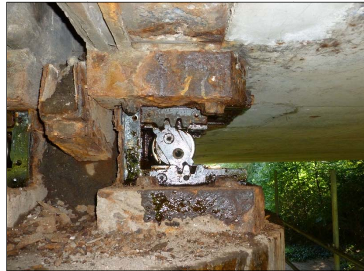
Bearing D2 – South Elevation
