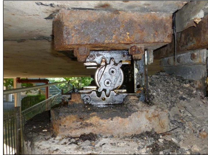
Bridge B1 – South Elevation
