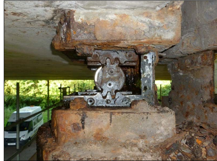
Bearing A2 -North Elevation
