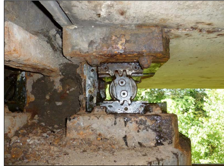
Bearing D1 – North Elevation
