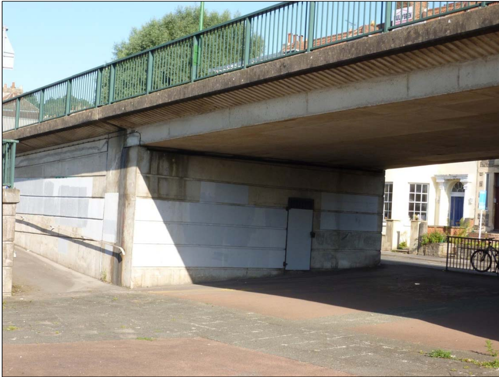
CABOT WAY – ABUTMENT
