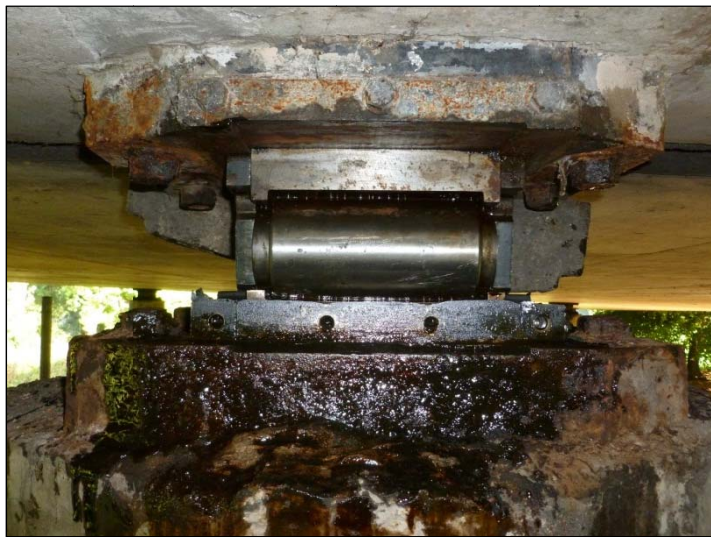
Bearing C2 with Grease Box Removed
