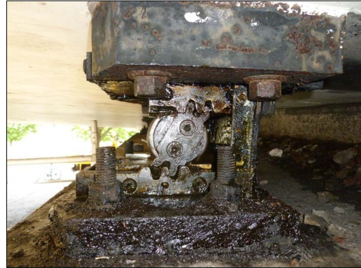
Bearing C – South Elevation
