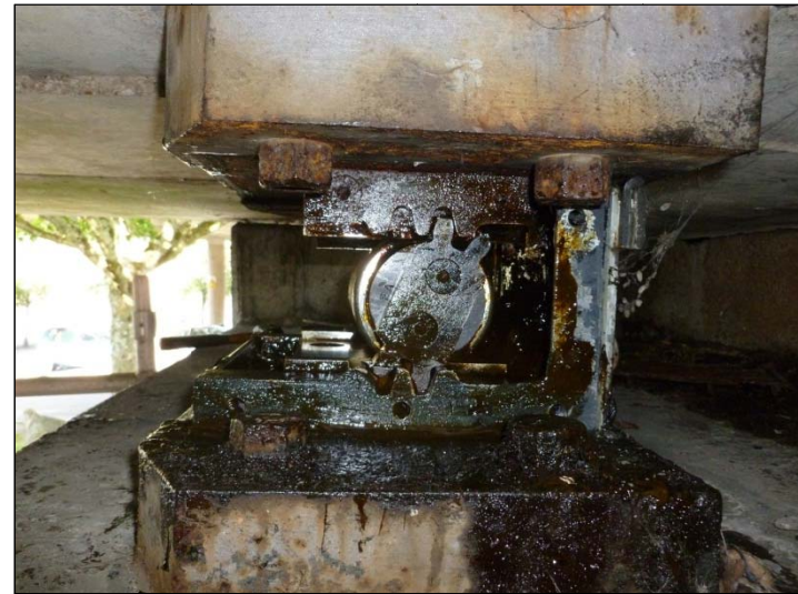
Bearing A – South Elevation
