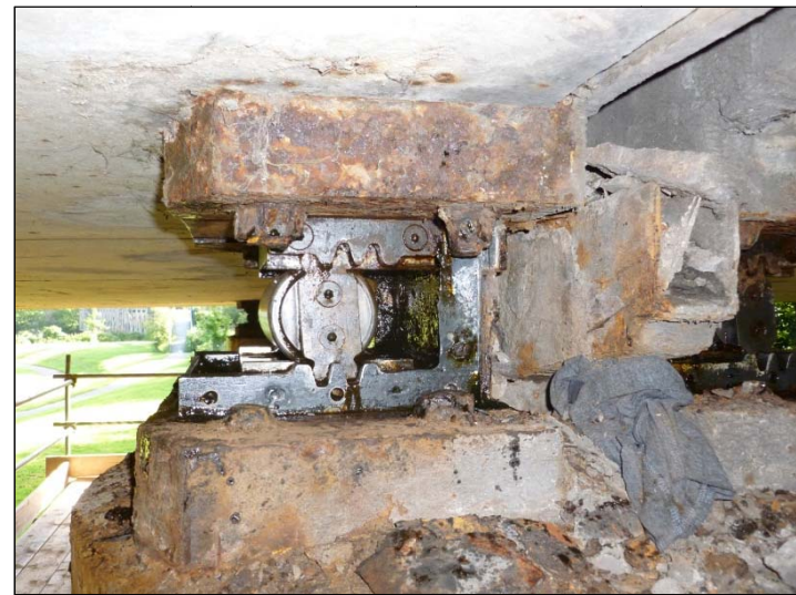
Bearing B1 – South Elevation
