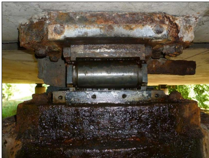
Bearing B2 with Grease Box Removed
