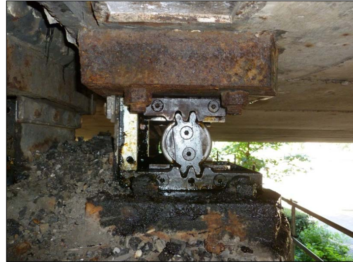
Bearing B2 – South Elevation
