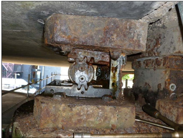
Bearing A2 – North Elevation
