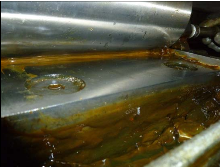
Bearing A; The base plates and fixings are in good condition.
