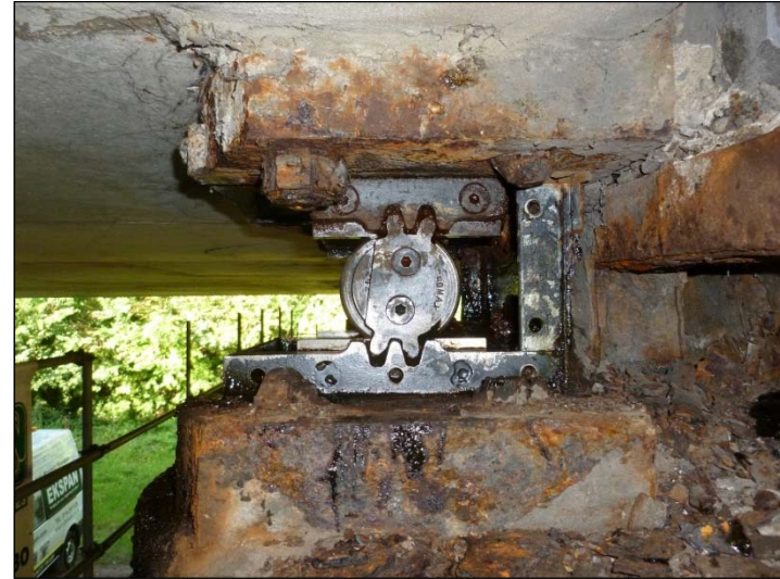
Bearing B2 – North Elevation
