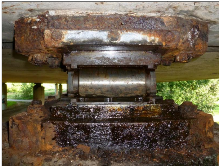
Bearing A2 with Grease Box Removed
