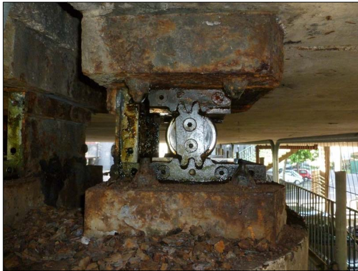
Bearing A1 – North Elevation
