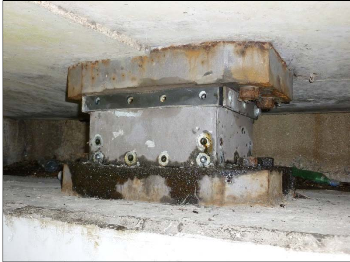
Bearing A – Before Removal of Grease Box
