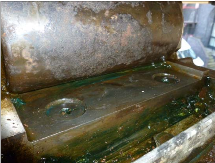
Bearing C1; Base plate and fixings are in good condition.
