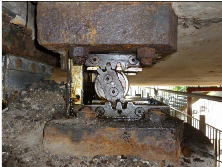
Bearing B1 – North Elevation
