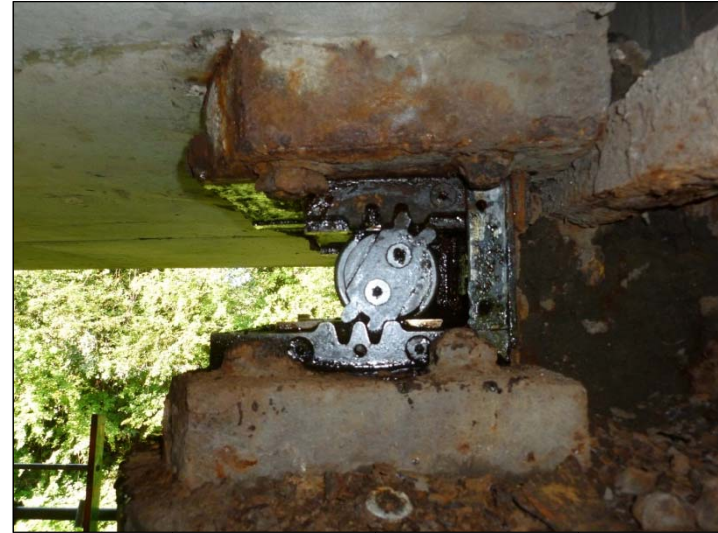
Bearing D2 – North Elevation
