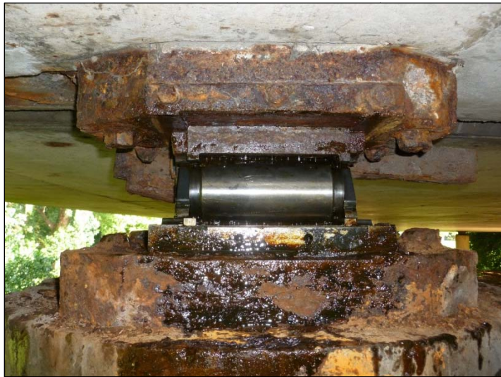
Bearing D2 with Grease Box Removed
