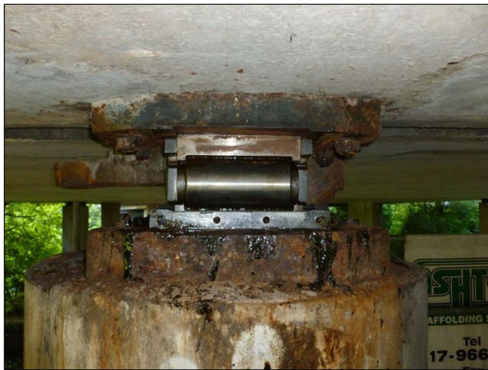
Bearing B1 with Grease Box Removed
